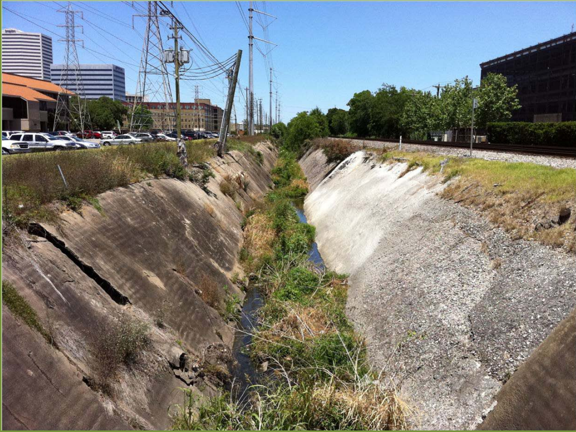
Failing concrete side slopes along the drainage ditch formally identified as W129-00-00 have caused erosion and have affected the integrity of the infrastructure.
