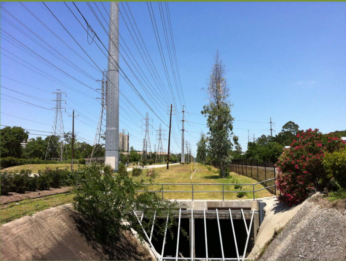
The W129-00-00 drainage ditch will be enclosed in dual 12-foot by 10-foot reinforced concrete boxes, as shown in this stretch spanning from Buffalo Bayou to San Felipe Street.
